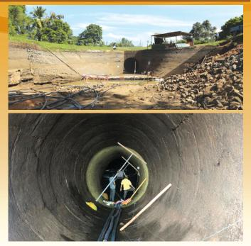
One of the most important major structures in the Right Bank (RB) Main Canal of the Udawalawa Scheme is the Siphon structure which is situated between the chainages 3 + 950 km to 4 + 330 km. The Udawalawa Scheme was constructed by the River Valley Development Board in 1963, and later in 1982, Mahaweli Authority of Sri Lanka (MASL) had taken over the
